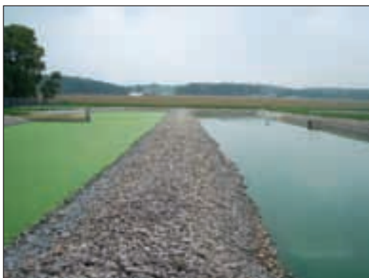
Picture of the two rock filters side-by-side, the one on the left has NO Grass Carp; the picture on the right is stocked with Grass Carp.
