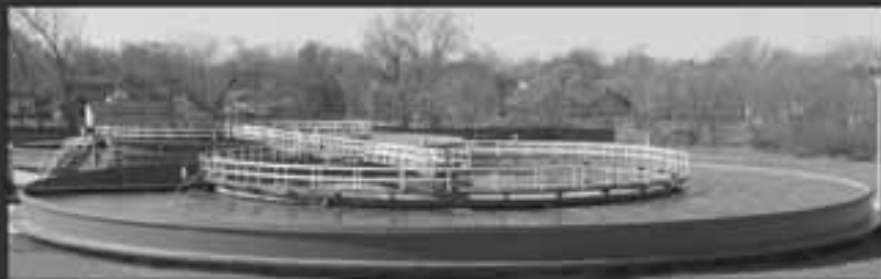
Wastewater Treatment Solutions
