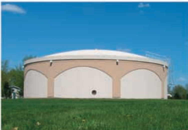
1.0 MG Natgun water tank for the City of Amboy, IL. Engineering by Fehr-Graham & Associates, Freeport, IL.
