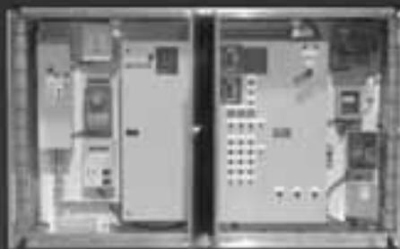
Pad Mounted Control Packages
